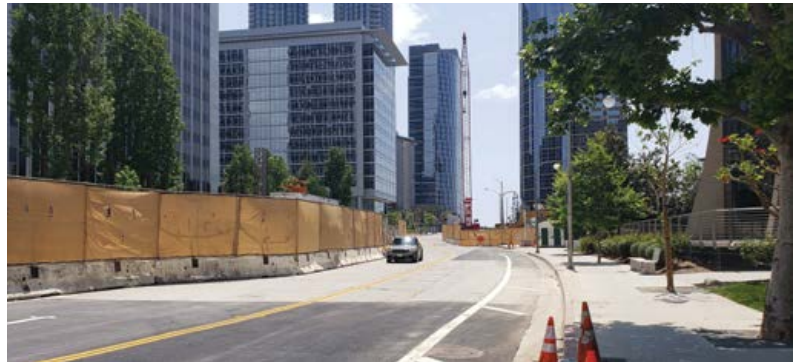
Street view of Constellation Blvd. looking eastbound from Century Park East.
